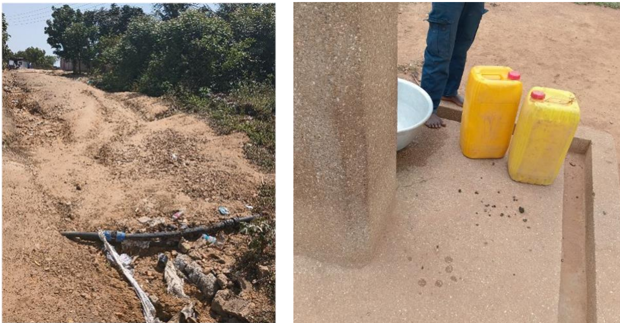
Image 2. Hazards observed during sanitary inspections related to exposed pipe in the distribution system (left) and animal feces at a standpipe (right).
