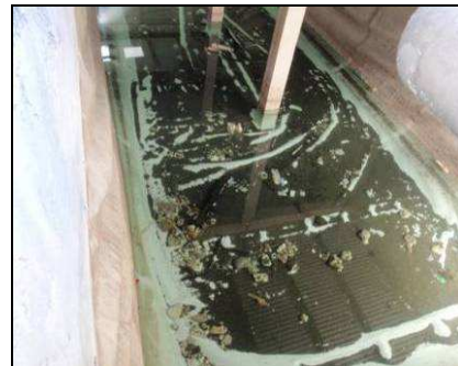
Unprotected water-storage
