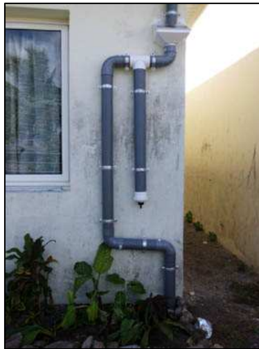
Improving safety of rain-water collection: Leaf-eater + first flush system
