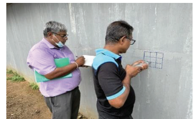
Figure 2: Rebound Hammer Test
